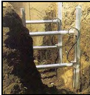
Vertical Hydraulic Shoring
